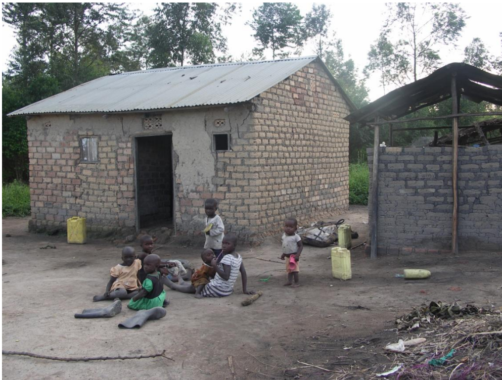
House in need of urgent repair ... windows needed and repair to cracks in the walls
